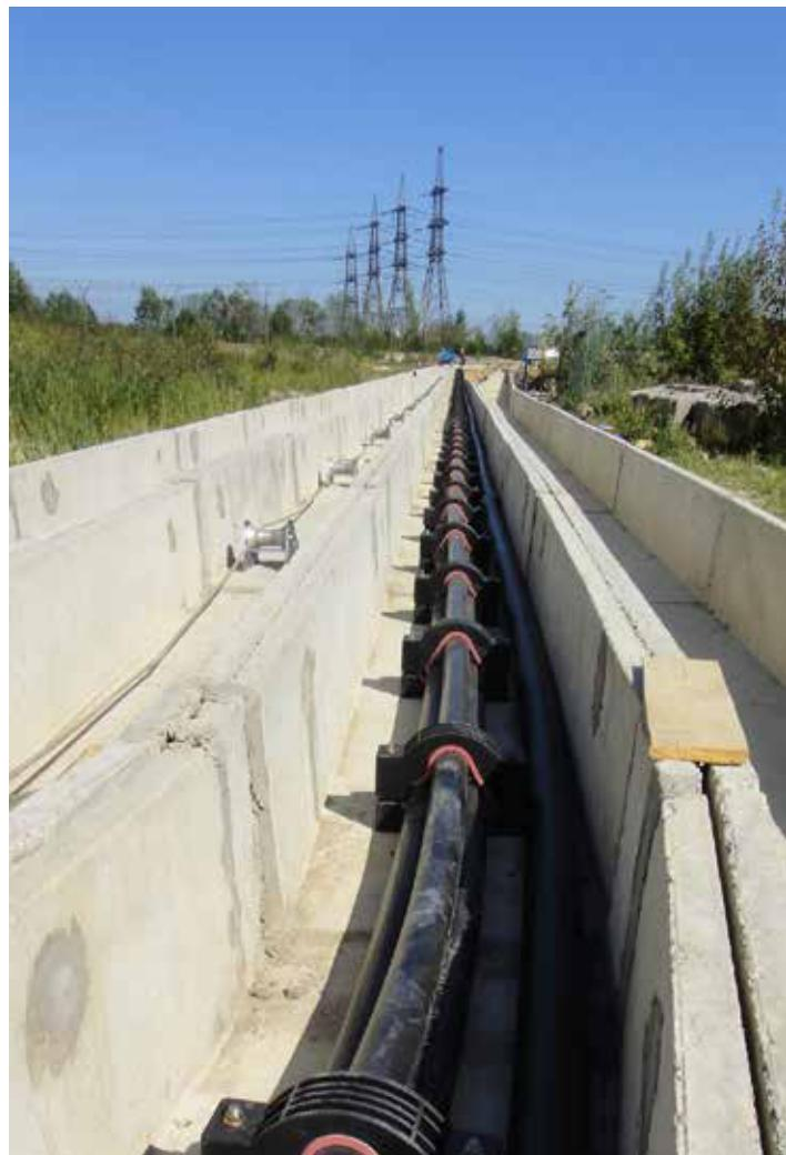
During XLPE 66-220 kV cable laying the bending radius should be not less than  $20xD$ , where  $D$  – outside cable diameter. When cables accessories installation is carried out with the use of a special template the preheating, minimal bending radius should be at least  $15xD$ .
